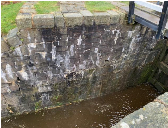
Completion photo showing leaks sealed
